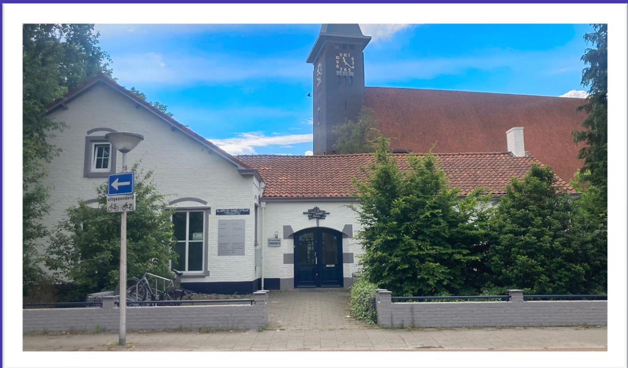
Valeo Primary School School Building
